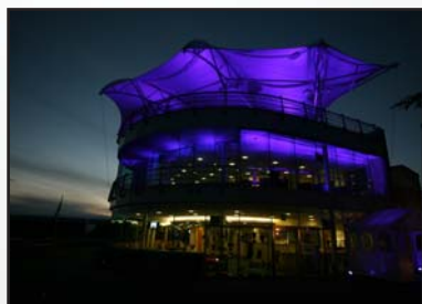
BRDC Clubhouse. First floor lit by Color Block 2 fixtures. © Jakob Ebrey
